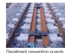
Derailment prevention guards
