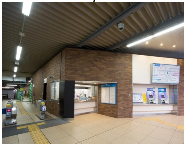
駅舎構築工事(世田谷代田駅) Station building construction (Setagaya-Daita Station)
