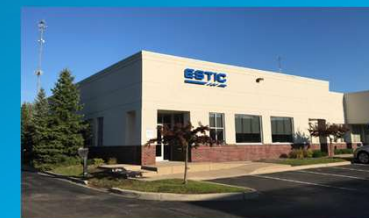
Novi Technical Center
