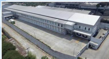
Cella Gemilang Logistik Warehouse (ナロゴン)
