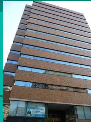
HQ's office in Osaka
