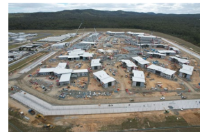
Southern Queensland Correction Centre
